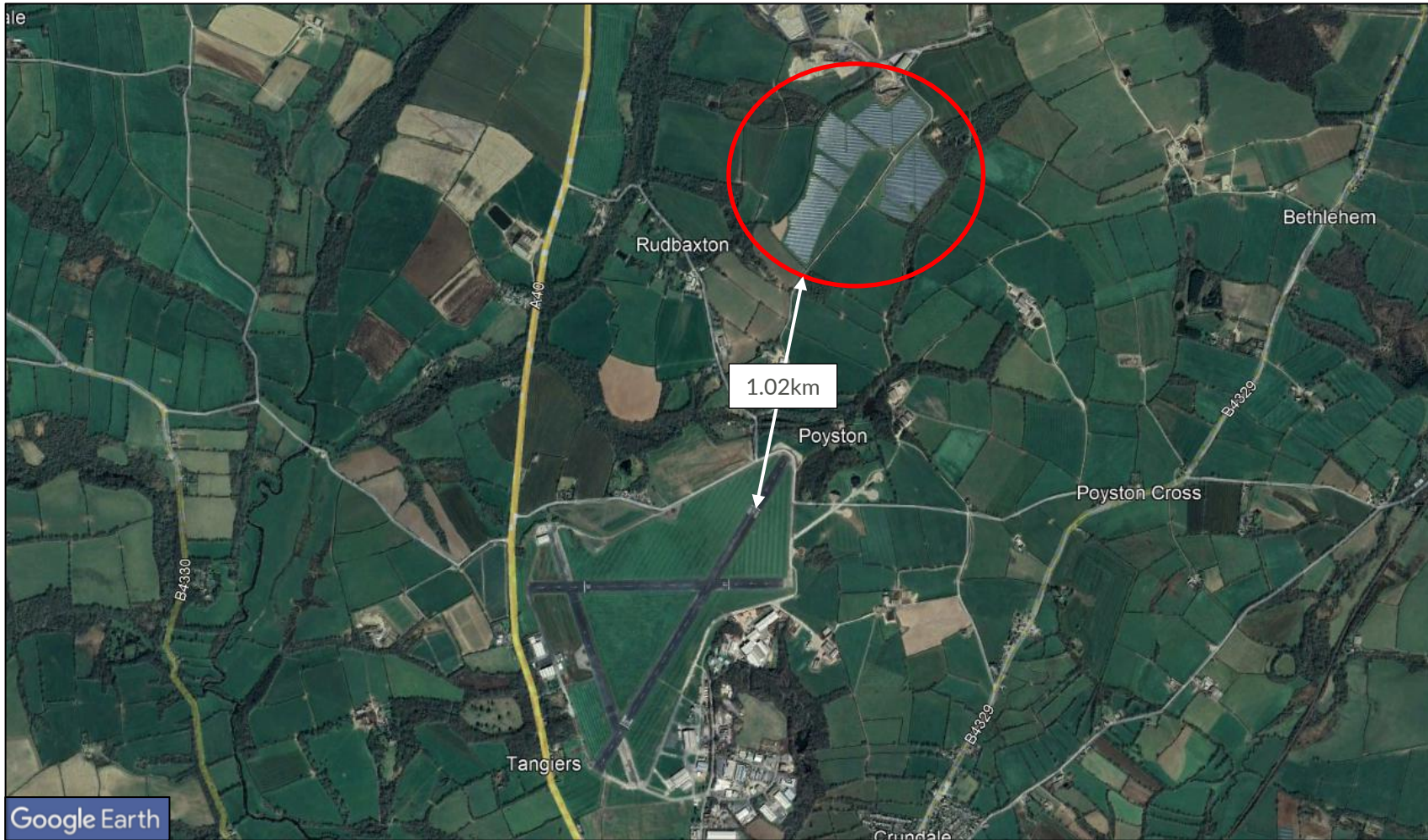
Figure 8 Existing solar PV development on the approach to Haverfordwest Airport
