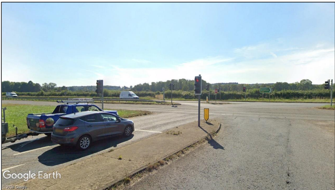
Figure 4 View of the road intersection directly south of the runway 01 threshold
